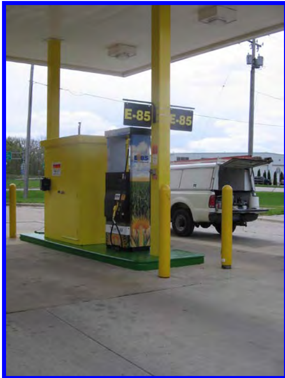
Permanent station with below ground tanks
