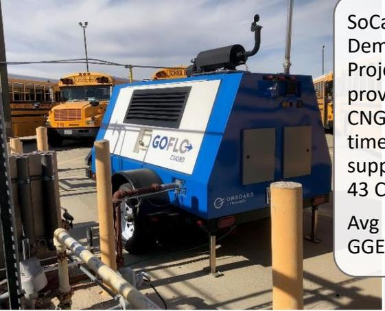
SoCalGas 2<sup>nd</sup> Demonstration Project. GoFlo® is providing additional CNG capacity for a time-fill station supporting a fleet of 43 CNG school buses.
